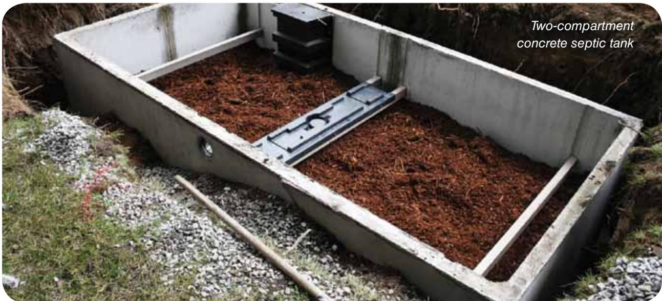
*Two-compartment concrete septic tank*
